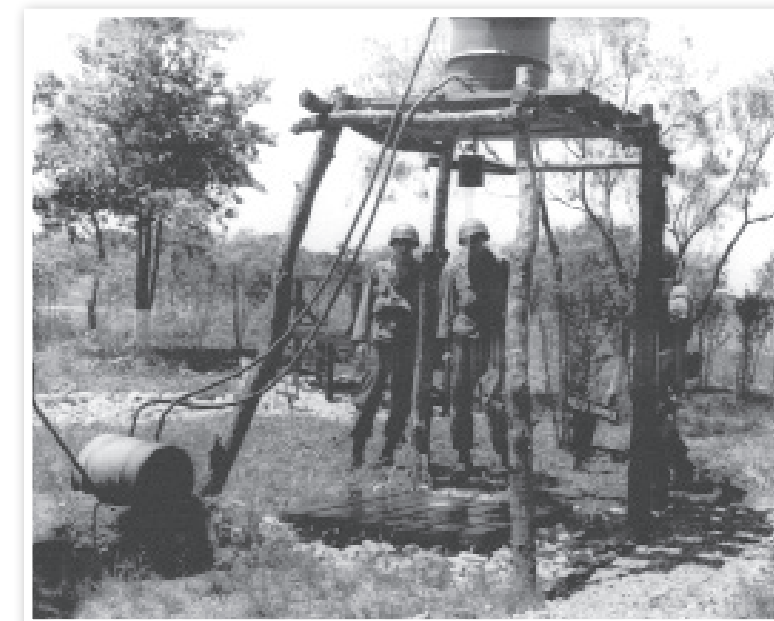
A field shower constructed from fuel drums
